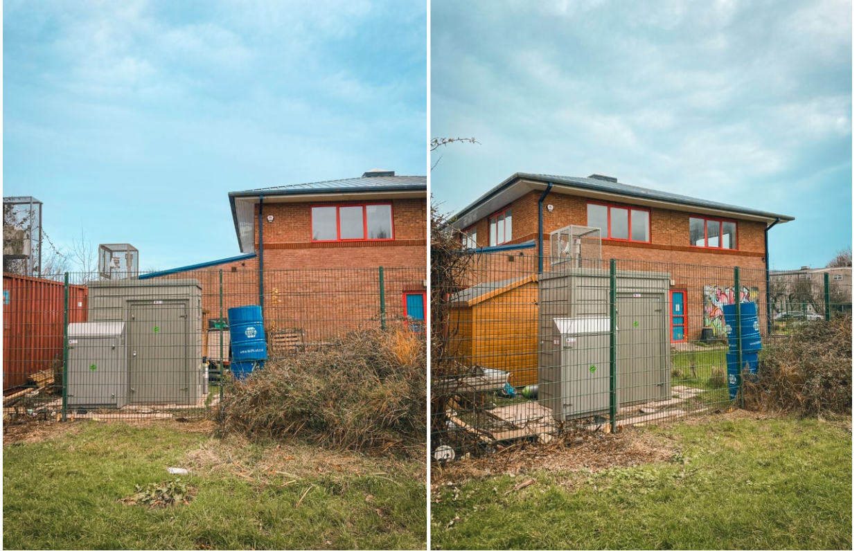
Figure 2: Eastbourne, Cabin Upgrade.
