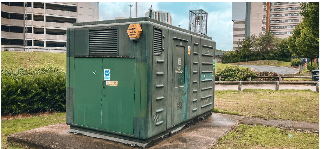
Figure 3: Leeds Centre, existing cabin to be upgraded.
